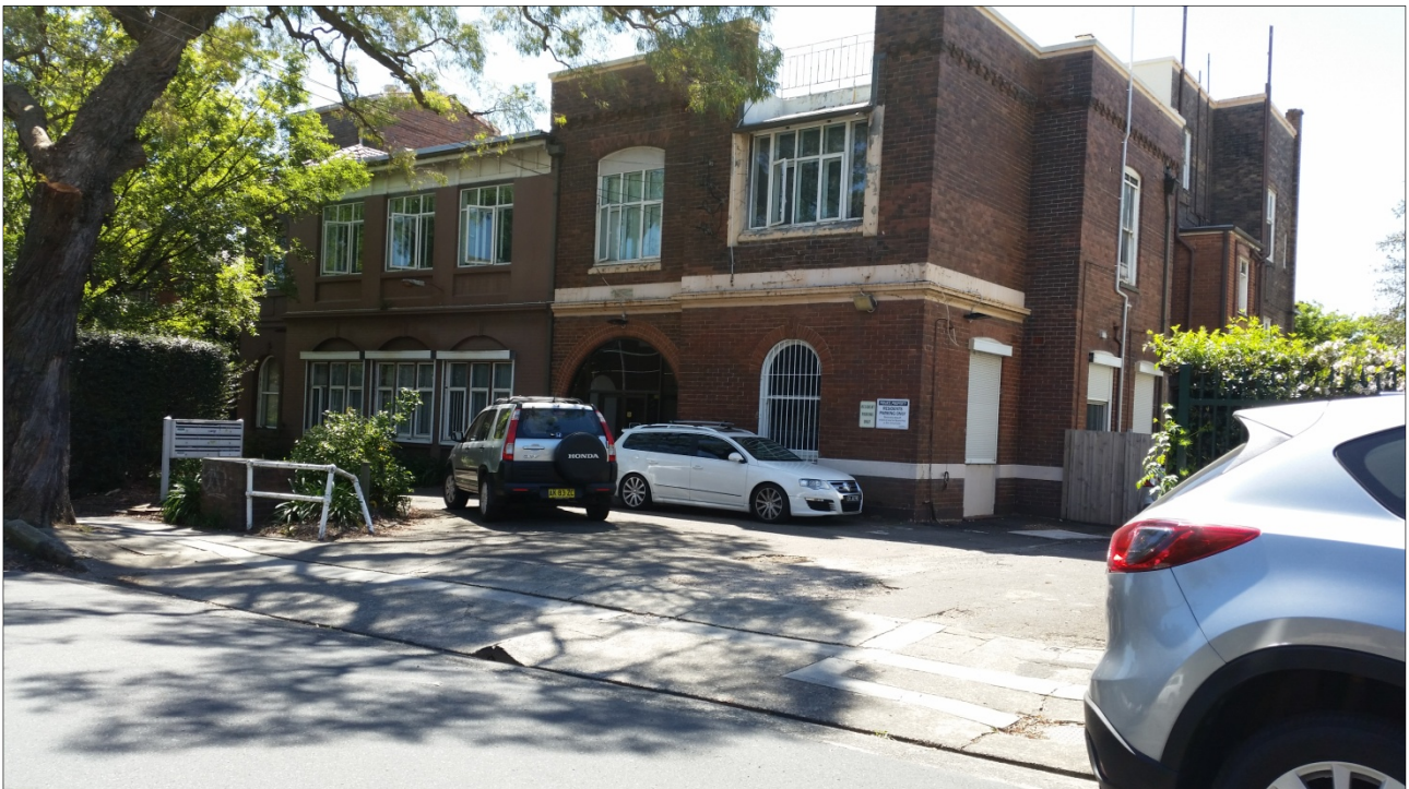
Image 3: View of Mary Andrews College building (formerly the Braeside Private Hospital) as viewed from Cambridge Street.
