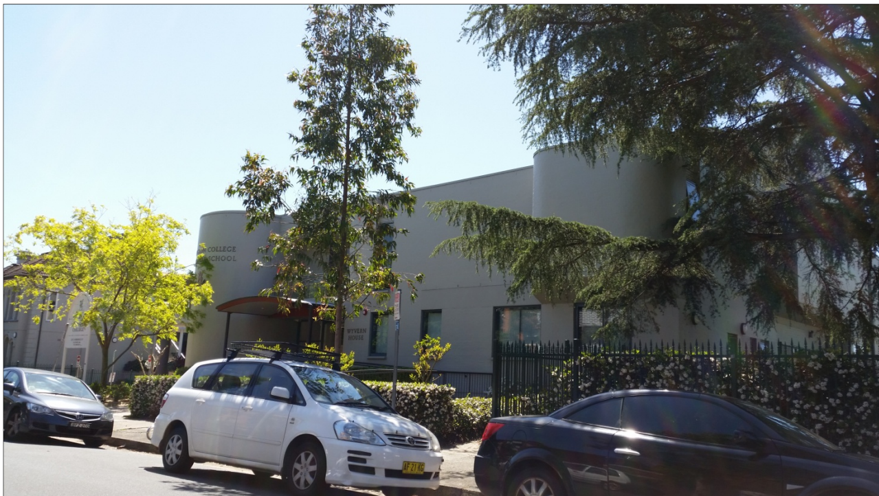
Image 8: View of the Wyvern building as viewed from Cambridge Street.
